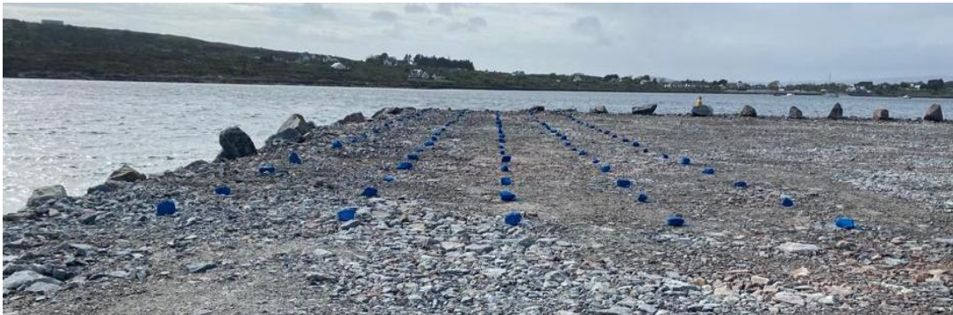
Figure 3 -Drilling Pattern laid out
