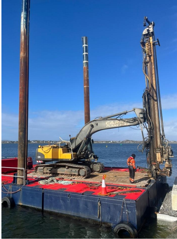
Figure 8 - Drilling Rig on Barge
