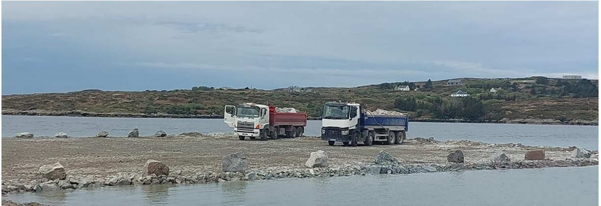
Figure 2- Blasting Platform 1 & 2 Being constructed
